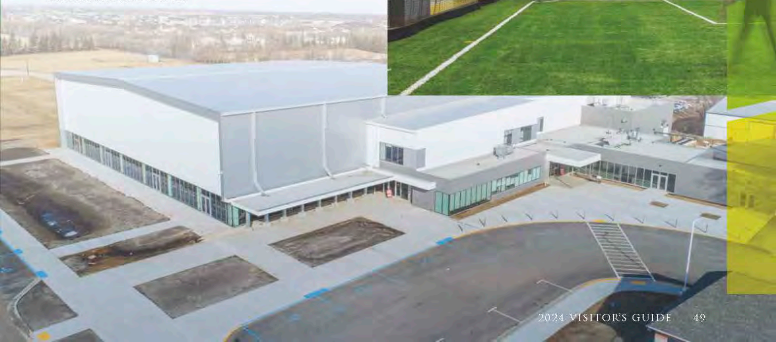
Meridian Exhibition Centre – Aerial View
